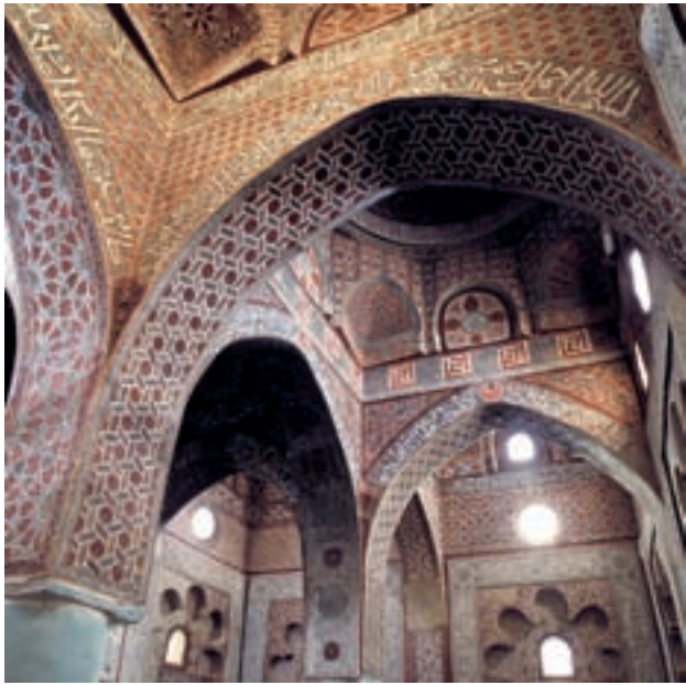
Fig. 5 Madrasa Amiriya, Radà, Yemen. A view of the prayer hall after conservation.
